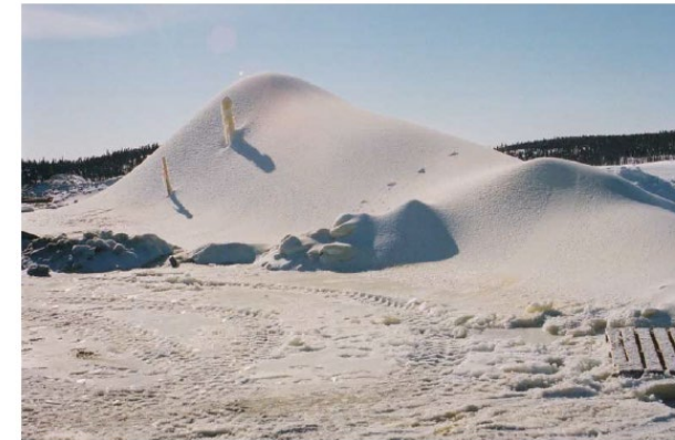
Fig. 2. Spray ice mound after completion.
